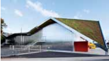
Multi purpose sports hall Lisieux (14) built
