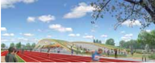
New outdoor sports track and field, stand and table tennis hall Marcel Guillot Le Neubourg (27) 1st phase built, 2nd phase due 2013
