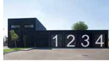
Offices and light industrial units for BURLOLOC Tremblay-en-France (93) built
