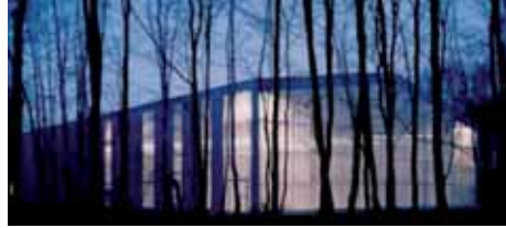
Sports Complex - Gymnastics Hall Jean Guimier Tremblay-en-France (93) built
