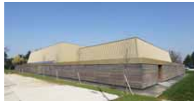
Sports complex and outdoor sports fields Les louvrais Pontoise (95) built
